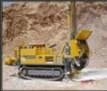
Photo: Core drilling machine drills through limestone deposits at a project in Iraq.
