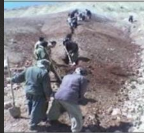
Photo: Trench sampling during the preliminary exploration for a project in Iraq.
