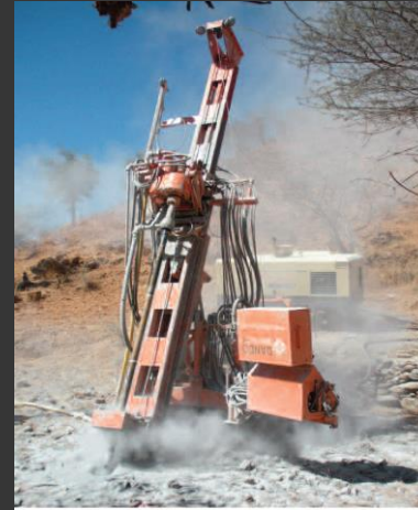
Mintec 6 Rotary Drilling Rig
